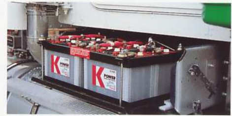
BATTERIES UNDER CAB
