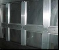
Back wall constructed with interlaced stamped and extruded hat section grid
