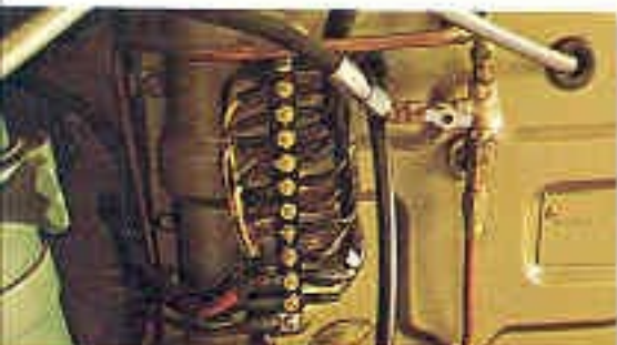
13. Piping & wiring—the most modern used in trucks today. The tubing and cable are positioned cleanly, easy to get at.
