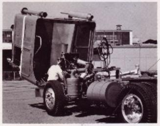
Reduce service costs with Kenworth's easily operated tilt cab, tilting to 75 degrees. Aluminum liner over engine compartment facilitates cleaning.
