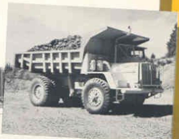
**TELESCOPIC HOIST** is Kenworth-patented. Fast action both up and down is assured by this single acting, two cylinder, straddle mounted, three stage hoist. Easily removed for service with truck loaded or unloaded. A single-lever, three-position hoist control
