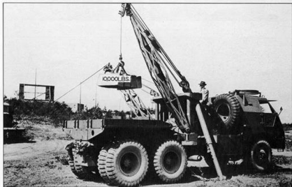
Testing the twin-boom Holmes equipment on the Kenworth. Note the M1 heavy wrecker in the background: a Kenworth 572; this was the only M1 type with full-power crane (100 produced, 1943).
