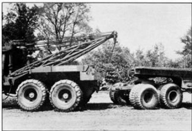
When tested with a dolly adaptor (turning a semi- into a full-trailer) it was found that the rig would all too easily jack-knife when attempting to reverse.
