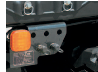
Test connections on compressed-air brake system.
